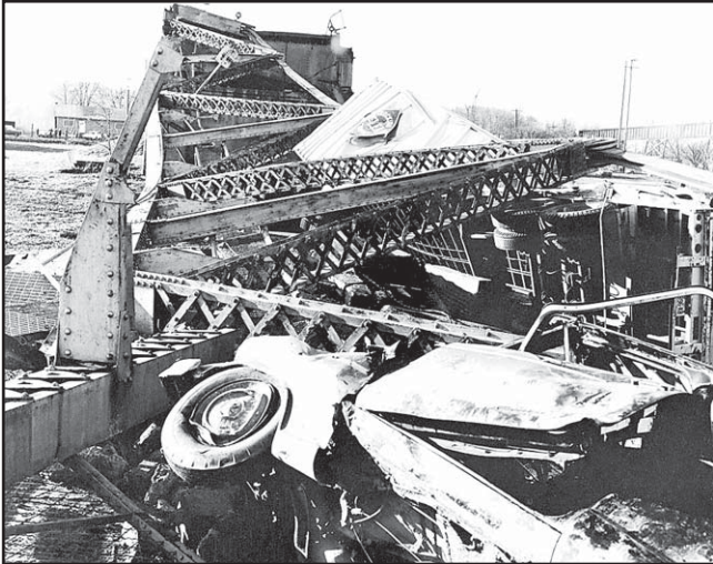
Dec. 15, 1967: The Silver Bridge at Point Pleasant collapsed, killing 46 people. The Silver Bridge was built by the American Bridge Company of Pittsburgh and opened to traffic on May 19, 1928. The accident led to the passage of legislation for a national bridge inspection and safety program.
