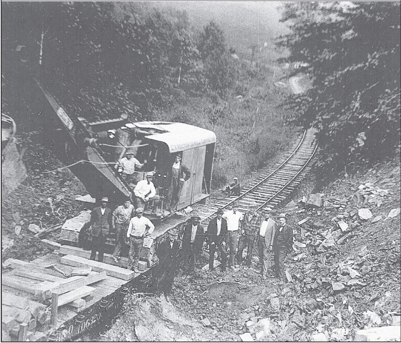
Road Construction... Building the road between Sutton to Flatwoods in the early 1930's was no easy task. A large mechanical shovel was the principal way to move large amounts of earth during that period. The reason for this photo and the people in it are unknown. The photo is courtesy of Craig A. Smith collection and is featured
