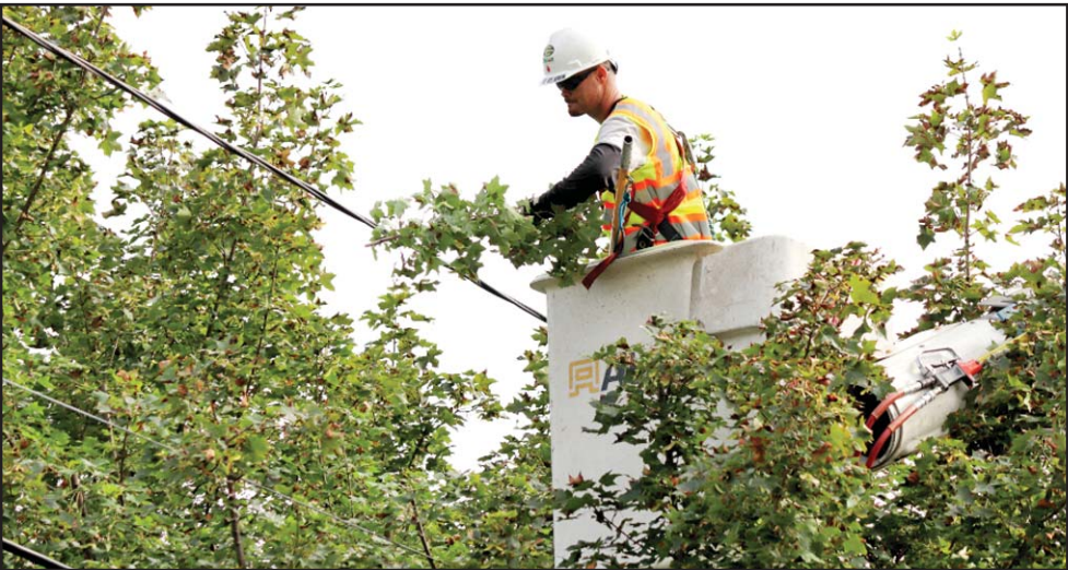
Utility personnel trimming trees near FirstEnergy power lines
